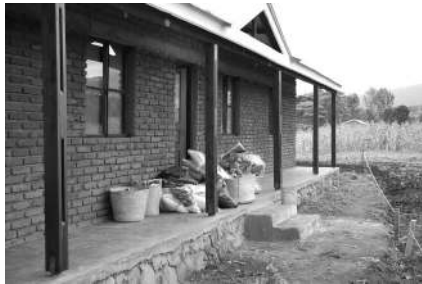
The first completed Young Men's House on move in day! The second Young Men's House is currently under construction.
